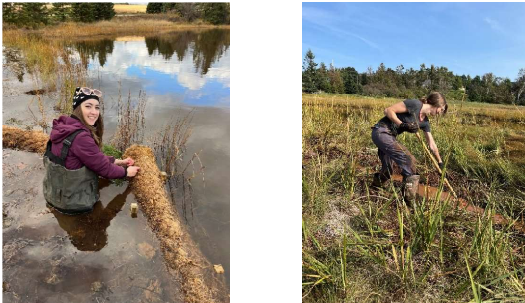
Figure 33. Executive Director Shayla Steinhoff digging runnels and installing coir
