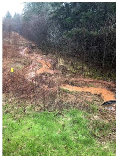
Figure 8. Silt run-off caught in large ditches after heavy rain fall to allow the silt to settle out of the water. In areas without management, this water carrying silt will run into our streams, damaging fish habitat.
